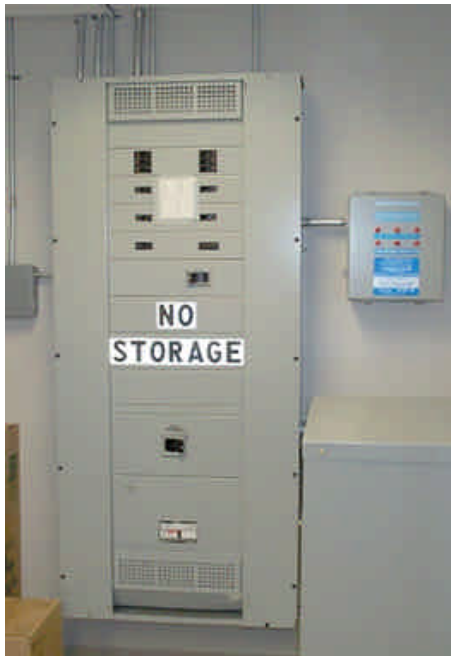
Figure 7. The 480-V distribution panel shown here feeds a 480V - 208Y/120-V transformer (lower right), the 277-V lighting circuit and the two air conditioning units. Connected to the 480-V bus at the right side of the panel is a 200-kA-rated TVSS that provides both line-ground and neutral-ground protection.
