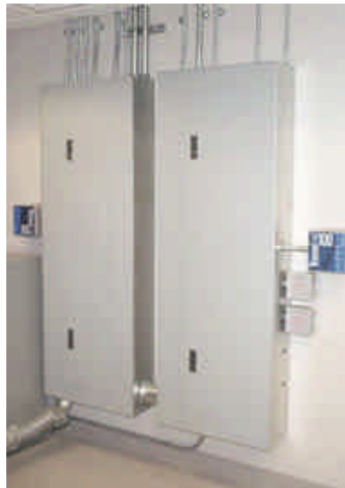
Figure 8. Two 120/208-V branch circuit panels supply the data center's computer room and other locations in the building, respectively. Each panel is protected by TVSSs rated at 100-kA (blue enclosures). Fire alarm and fire call circuits are additionally protected by TVSS devices rated at 20-kA. There are as many as seven layers of surge protection in critical portions of the data center's electrical system.
