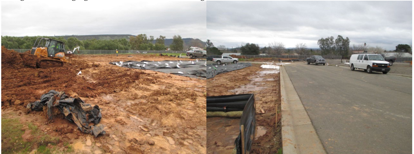
FEMA Site Development and Housing Assistance Project in Oroville, California March 2019
