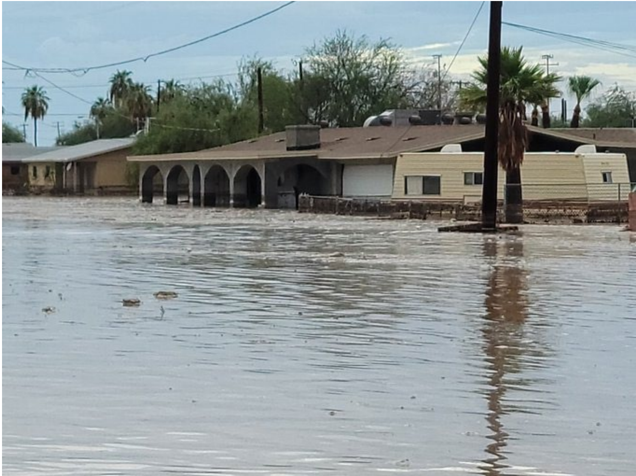
Figure 20 – Post-Flash Flood Photo in Gila Bend, AZ – 14 Aug 2021 (Photo courtesy of NWS)
